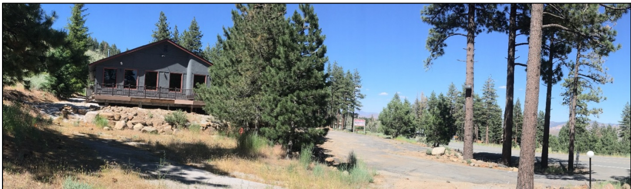
From south side of property, looking north at existing structure and parking lot (Mt. Rose Highway is on far right side of photo)
